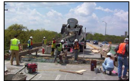
Picture of Bridge Joint Replacement over the Fox River
